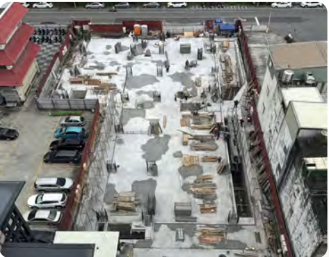
Concrete pouring of the B1 top slab of the new Hualien facility (aerial photo), April 20, 2026
